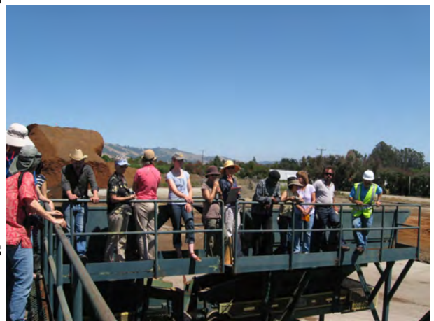
Sun Land Garden Products aerial walkway over conveyor system.
