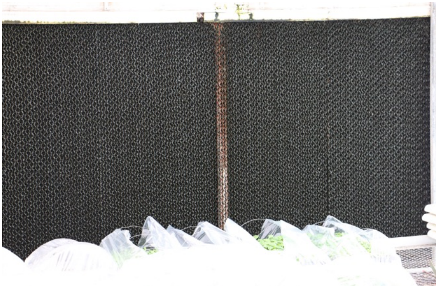
Left. The rear wall of the shade house. Water runs down the medium, and air passing through driven by fans to the front of the house, is cooled and flows through the shade house maintaining coolness and humid during hot days in summer.
