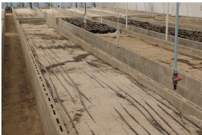
Left. Heating beds for seed and cutting propagation. The beds are filled with sand and hot water pipes regulated by a thermostat, keep the beds at the right temperature.
